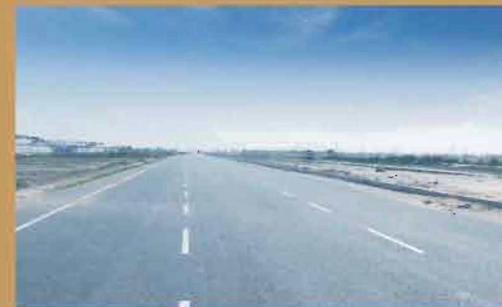
AN ACTUAL PHOTOGRAPH OF DWARKA EXPRESSWAY
