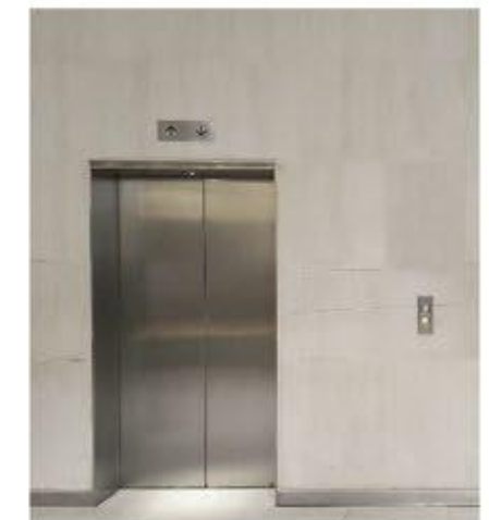
Common Area Maintenance
