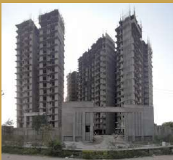
UNDER CONSTRUCTION SITE-2
