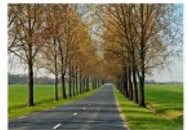
Internal WBM/Tar Roads
