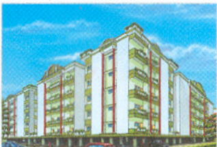
RESIDENTIAL APARTMENTS SR NAGAR
