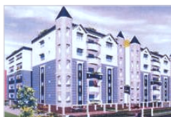
RESIDENTIAL APARTMENTS KONDAPUR
