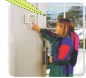
INTERCOM FACILITY WITH SECURITY DOOR
