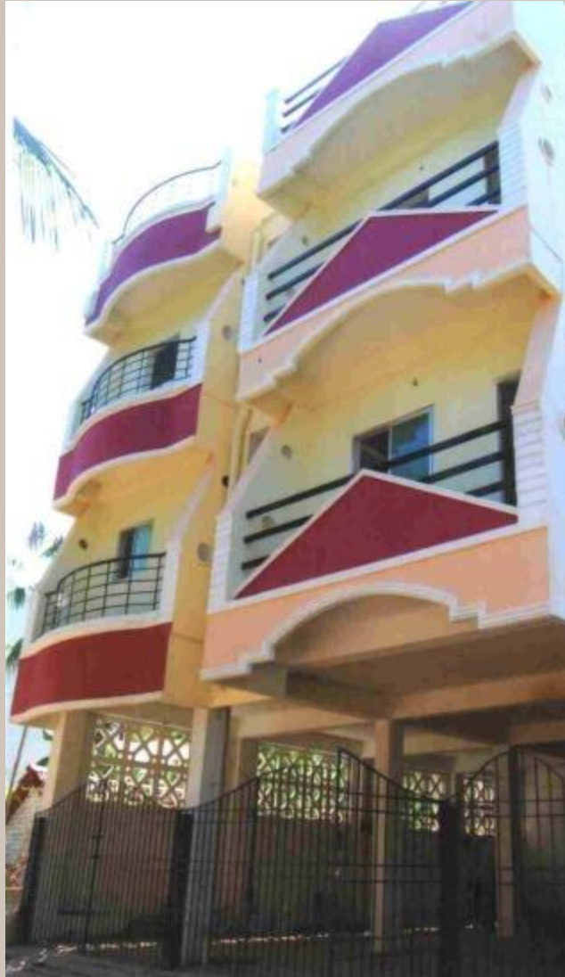
Diamond Building , Alandur
