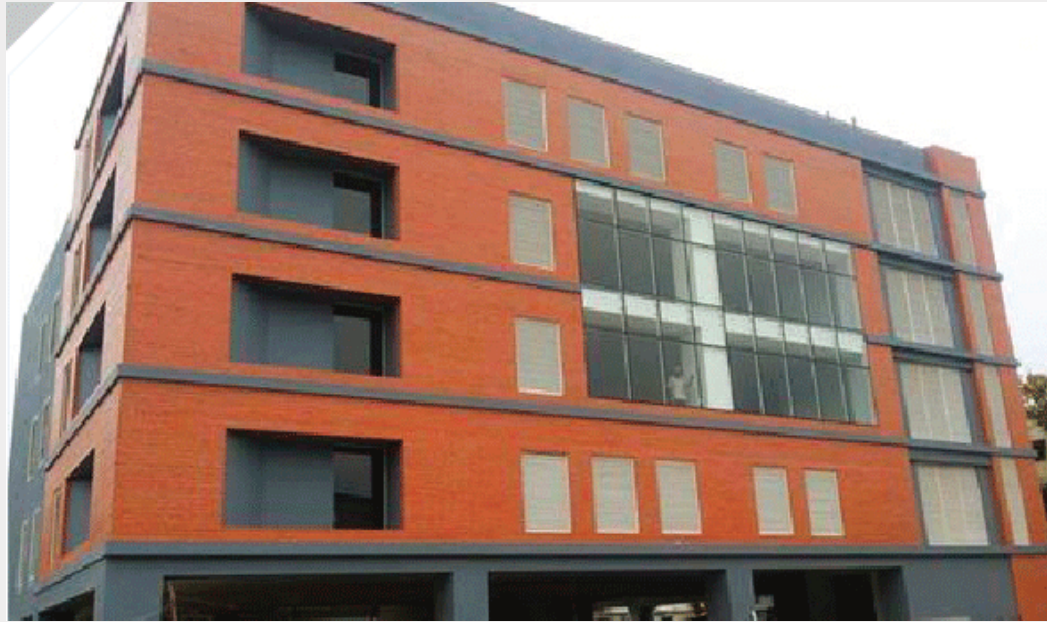
Kay Arr - Kodi 1 Tower Perungudi, Chennai
