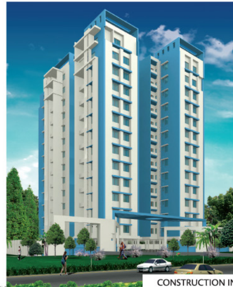
CONSTRUCTION IN FULL SWING
