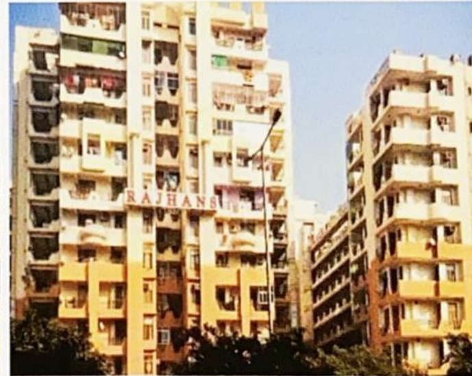
RAJHANS PREMIER APARTMENT, INDRAPURAM, GHAZIABAD
