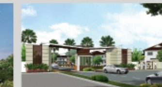
PEARL ESTATES Vidhani Circle, Mahal Road, Sitapura, Jaipur.
