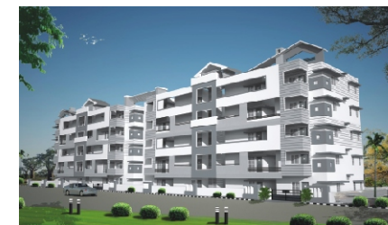
Forty East Facing Luxury Signature Apartments
