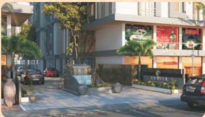
MAIN ENTRANCE GATE WITH SECURITY CABIN
