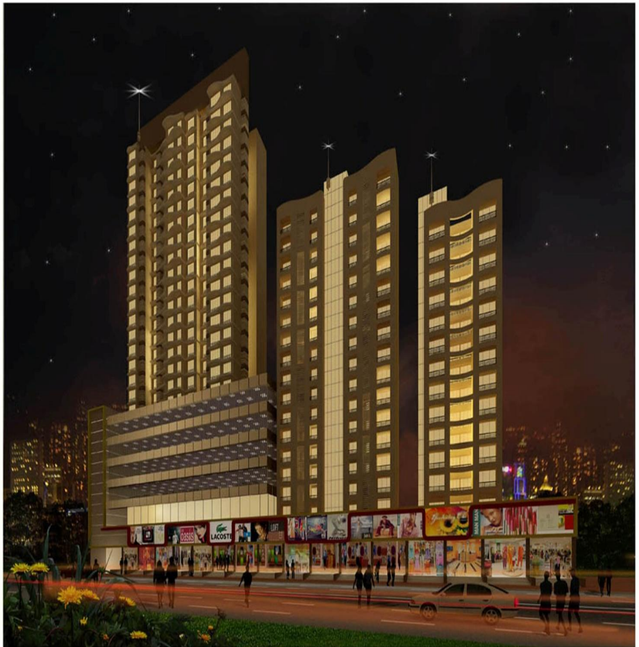
SHREEDHAM SPLENDOUR Main Link Road, near Lokhandwala Complex
