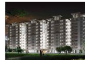
Metropolis, Jaisinghpura, Ajmer Road
