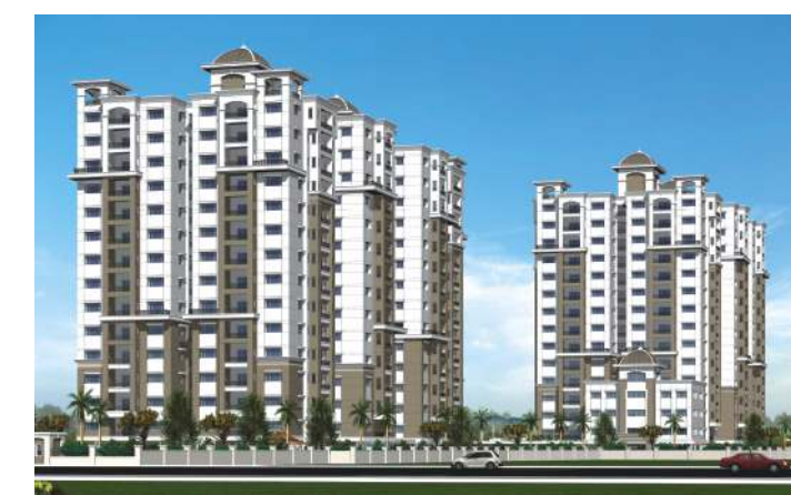
Fortune Towers, Hyderabad
