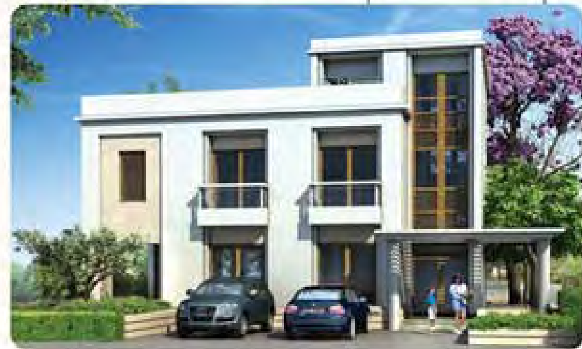
STREET SIDE VIEW
